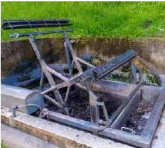
Installation of rotor screen for Grid removal of ETP
