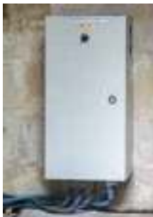
Inventor & electrical panels for water recovery system
